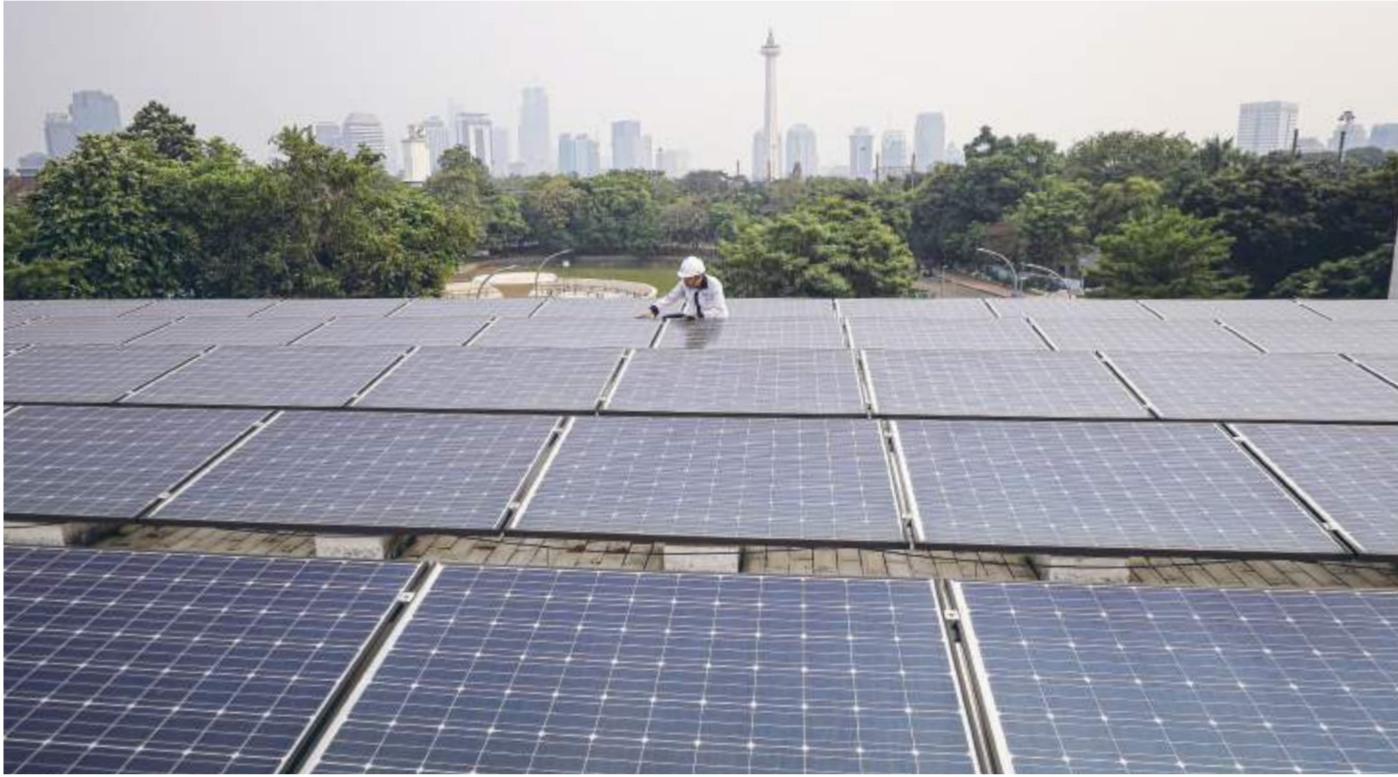
A maintenance officer checks the solar panels installed on the roof of the Istiqlal Mosque, Jakarta.
